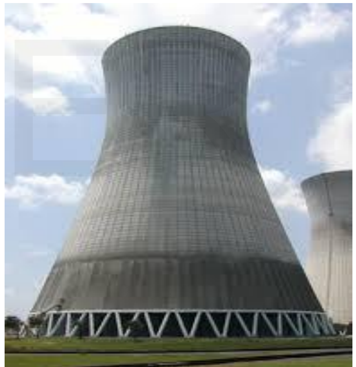
Figure 1: Natural Draught Cooling tower
